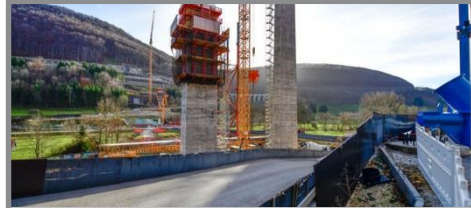
Building infrastructure e.g. bridges and locks, coastal defenses
