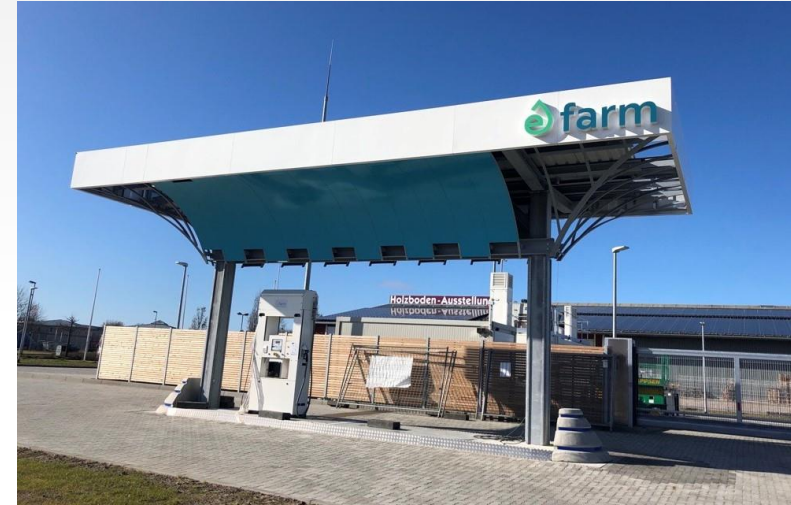
Hydrogen process: Building of a hydrogen filling station in Niebüll, efarm
