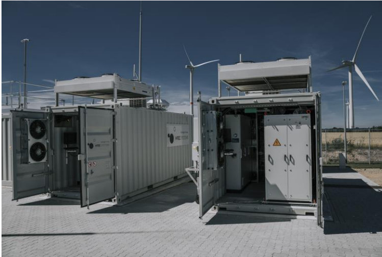
Hydrogen produce: Elektrolysis/compression at the wind park
